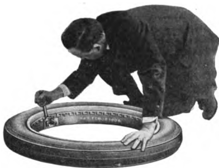
Fig. 6—Locking (or unlocking) the rim
